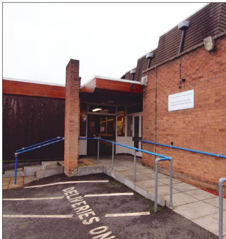
The existing Wingerworth Parish Hall which the Parish Council wants to replace
